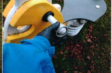
Finding: The end of handgrips and/or footrests have a cross Action: Monitor - No remedial work recommended section of less than 15cm2 and fail to meet the requirements of BS EN 1176 Part 6
