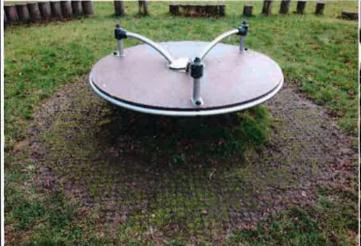
**Finding:** The height to the underside of the roundabout platform is less than 400mm and fails the requirements of BS EN 1176 Part 5
