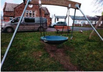
Finding: Swings of this design should have a secondary safety device fitted to prevent collapse of the seat in the event of a joint failure to meet the requirements of BS EN 1176 Part 2
